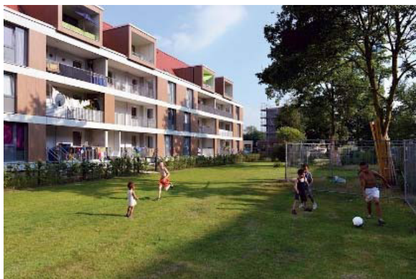
Εικ.60 The building after refurbishment with the added loggias
